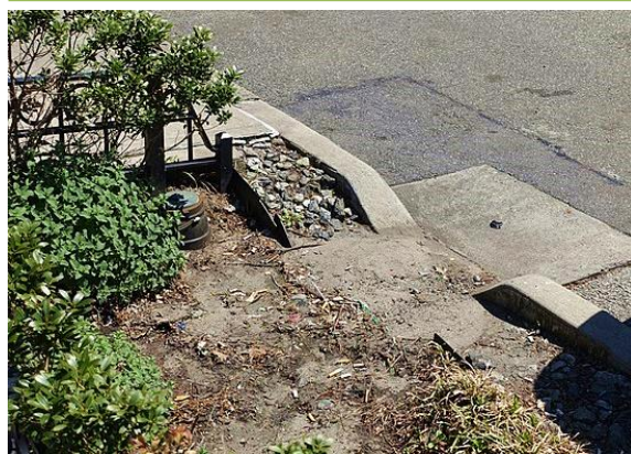
This new rain garden in a parking lot has gaps punched into the curb to allow water to flow in.
